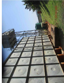
EXISTING 324kL WATER TANK
